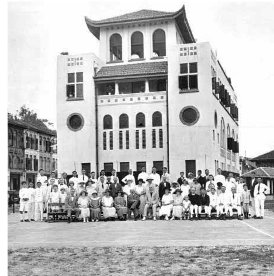
(Top) Denis Santry’s building plan of the proposed church and recreation rooms for the Telok Ayer Chinese Methodist Church, 1923. Building Control Division Collection, courtesy of National Archives of Singapore. (Above) Telok Ayer Chinese Methodist Church was consecrated by Bishop Titus Lowe on 25 April 1925. Designed by Denis Santry of Swan & Maclaren, it was a modern four-storey, concrete-frame building that was part-Byzantine and part-Chinese in design. Lee Brothers Studio Collection, courtesy of National Archives of Singapore.
